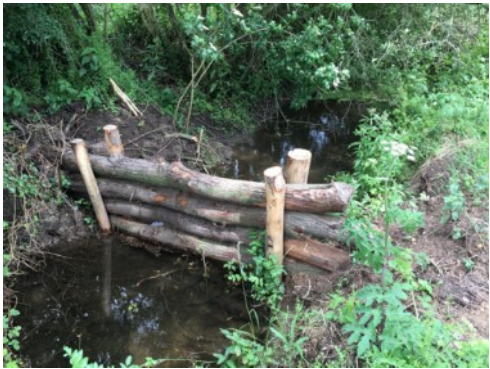
Example of a leaky dam
